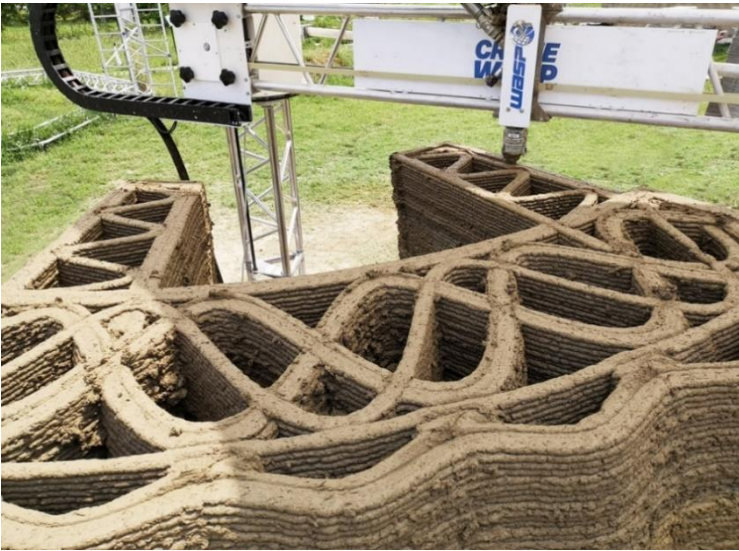
Figure 26: Italian company WASP has built one of the largest 3D printers in the world 125 . In the picture, the use of a clay-based 3D printer to build a sustainable house (“Tecla” project)
